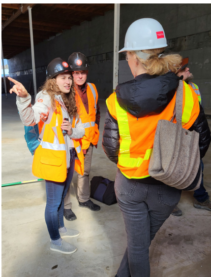
Francesca giving direction on the job site
