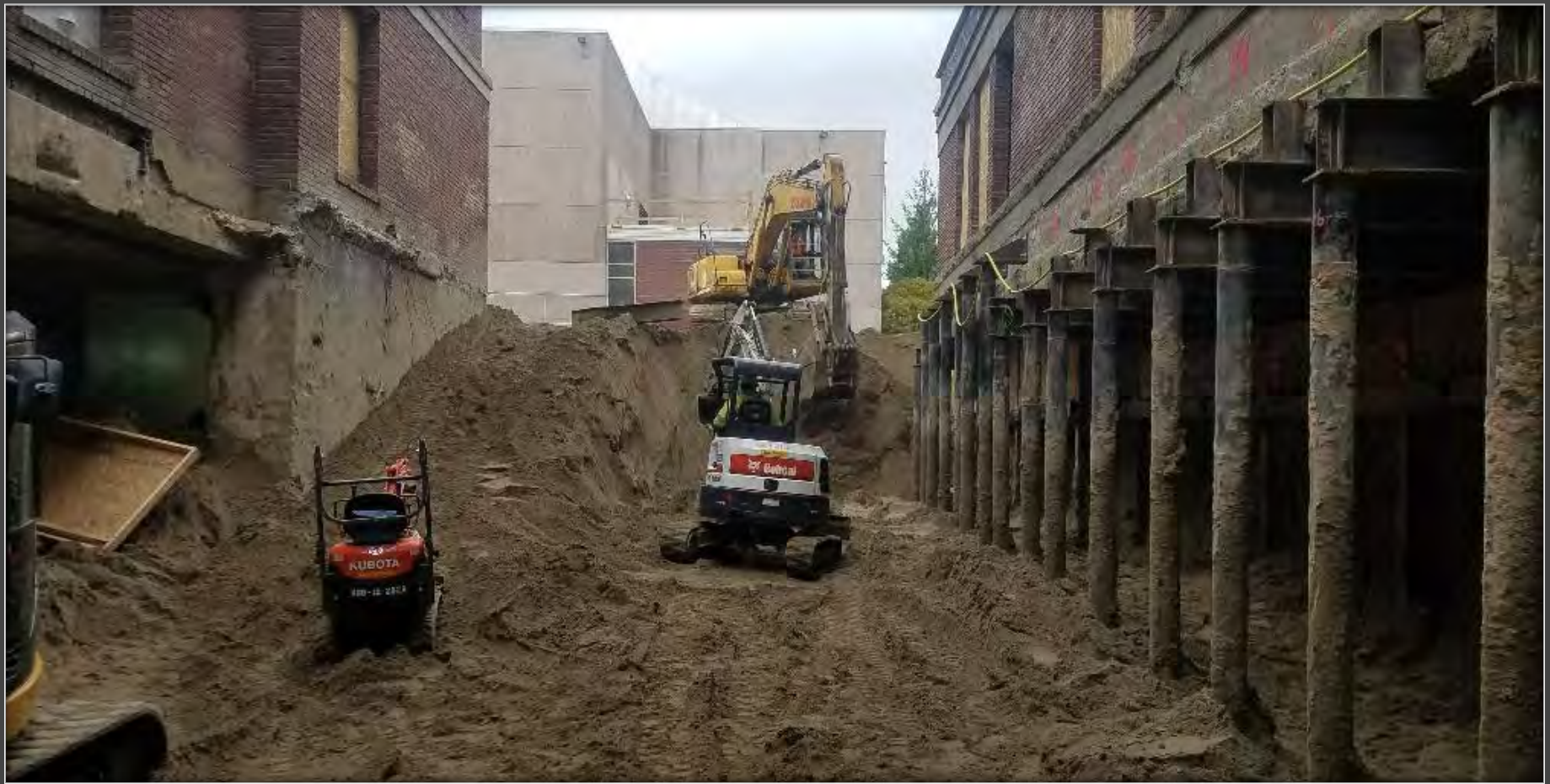
Excavation for 2nd lift of lagging
