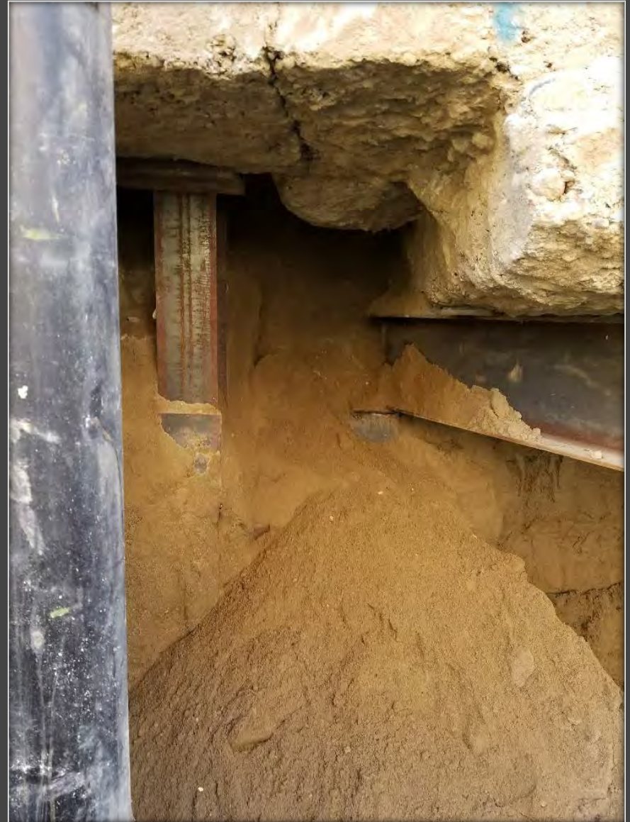
Angle bracket and spreader beam
