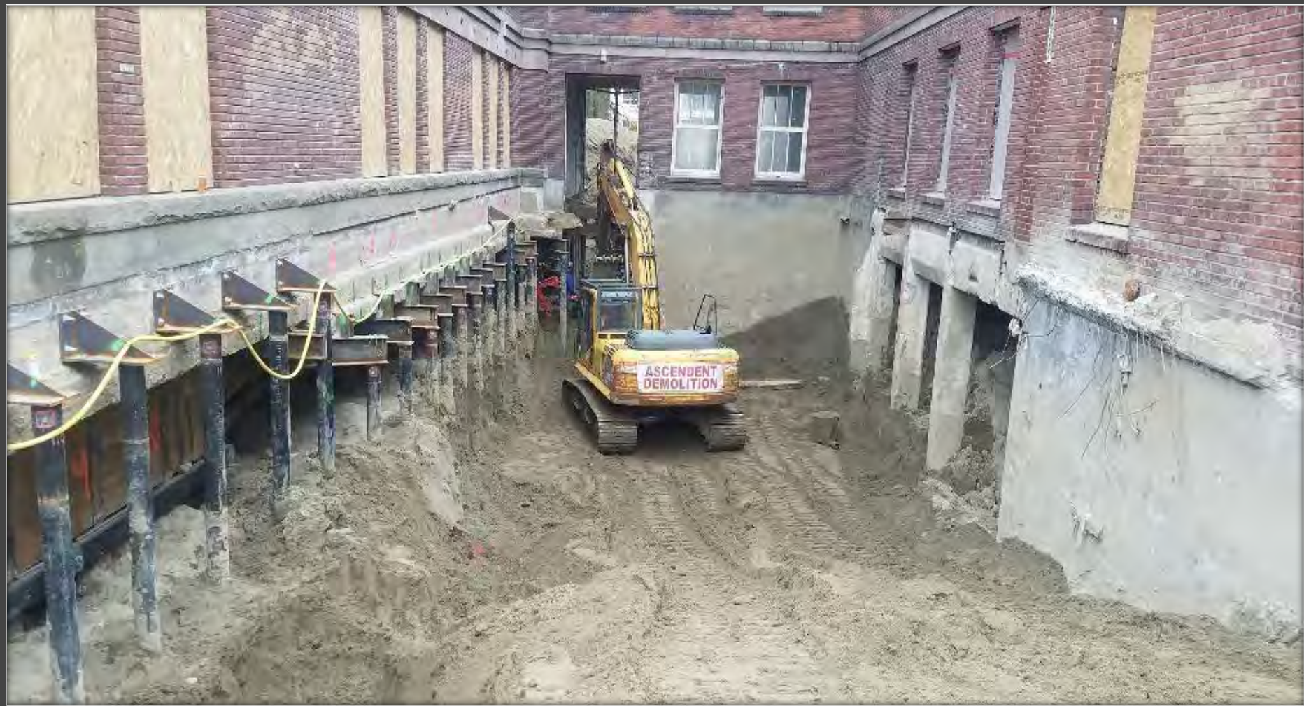
Excavation for 2nd lift of lagging
