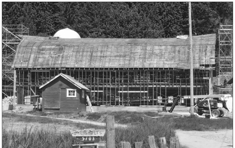
The Cooper Dairy Barn under renovation. Photo courtesy of Kirtley Cole.
