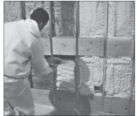
Spray foam insulation application.
