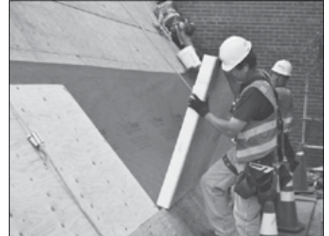
Installing structural insulated panels.
