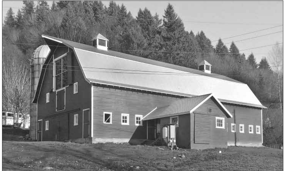
With grant funds from 4Culture and the Heritage Barn Preservation Initiative, the first phase of the Cooper Dairy Farm project, rehabilitation of the historic Cooper Dairy Barn, was completed in 2015.
